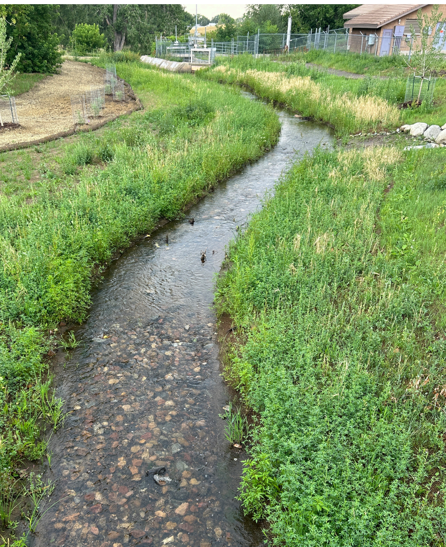
Stream improvements increased the flood capacity and allow for easier access to the creek.
