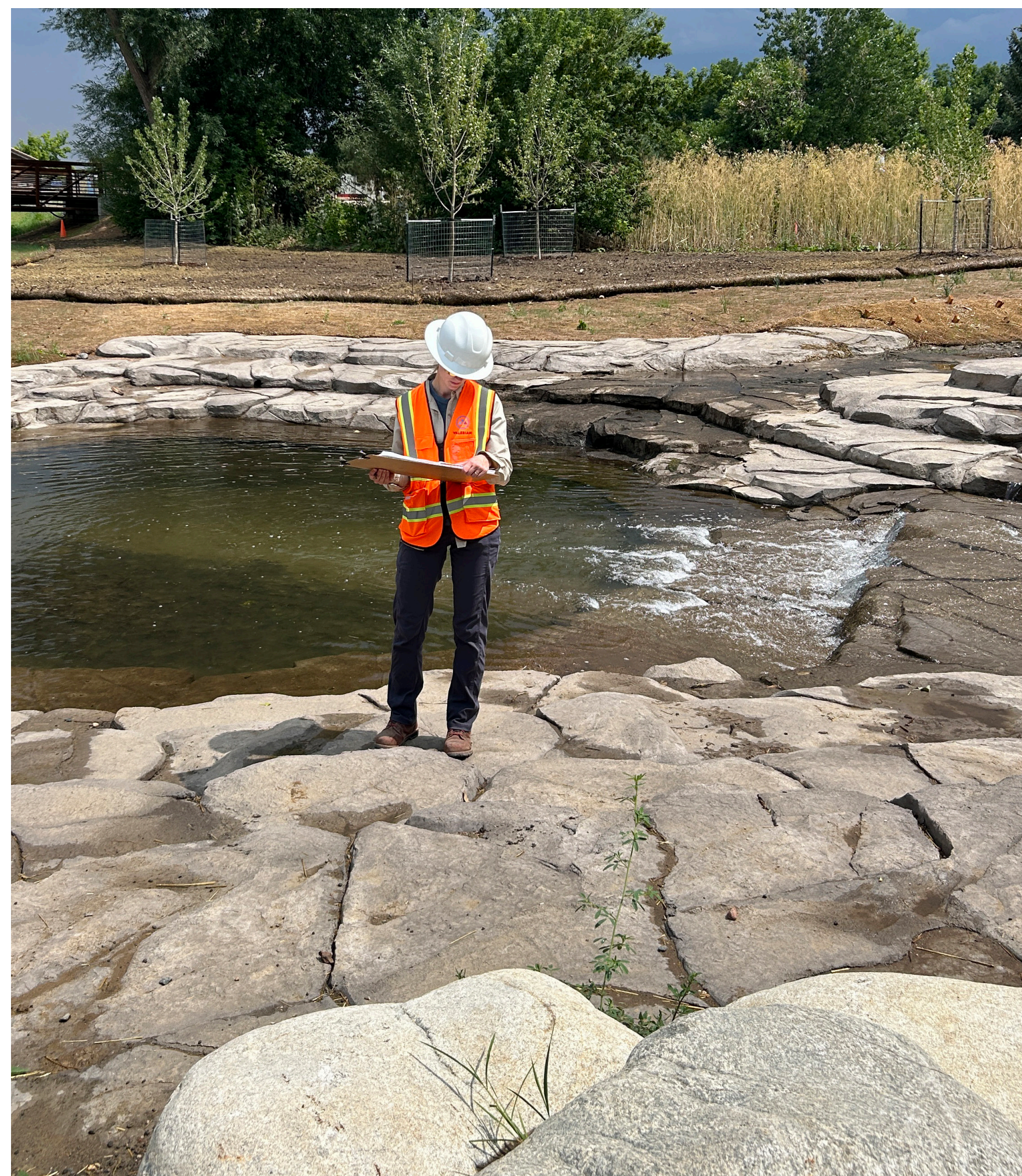
Stream structure mimics natural bedrock.
