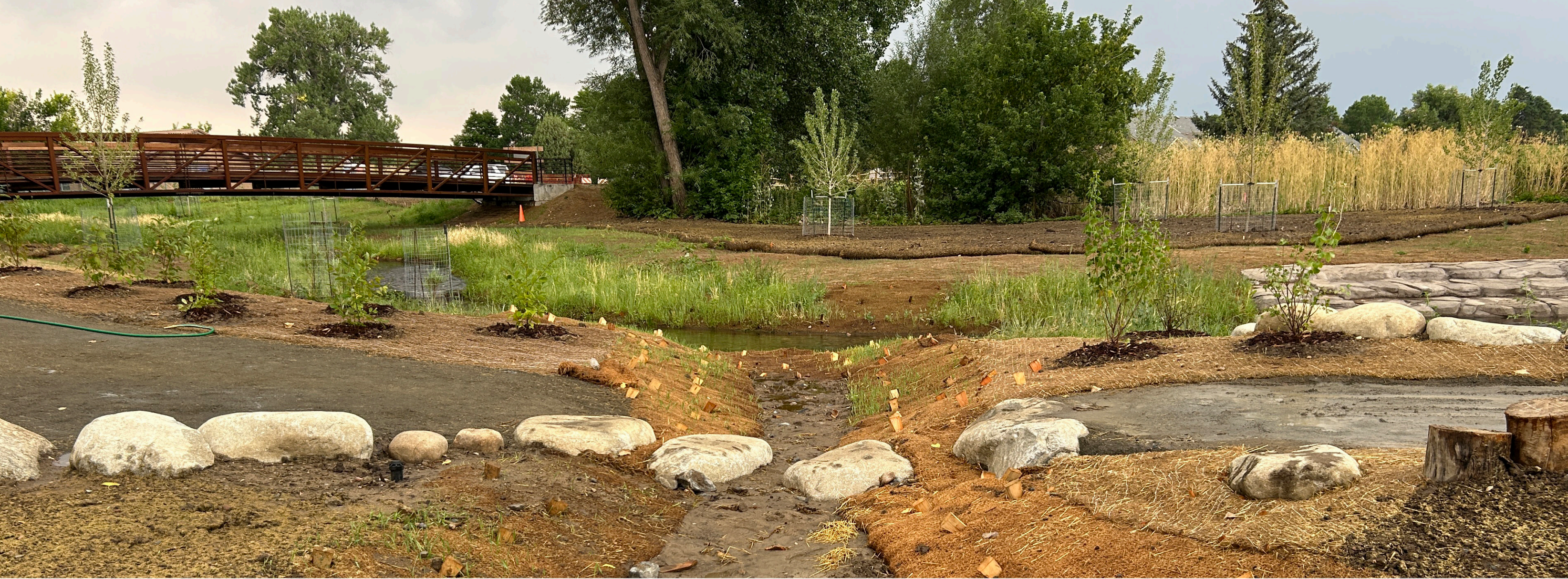
Boulders and logs installed to create natural play areas and improve stream access.
