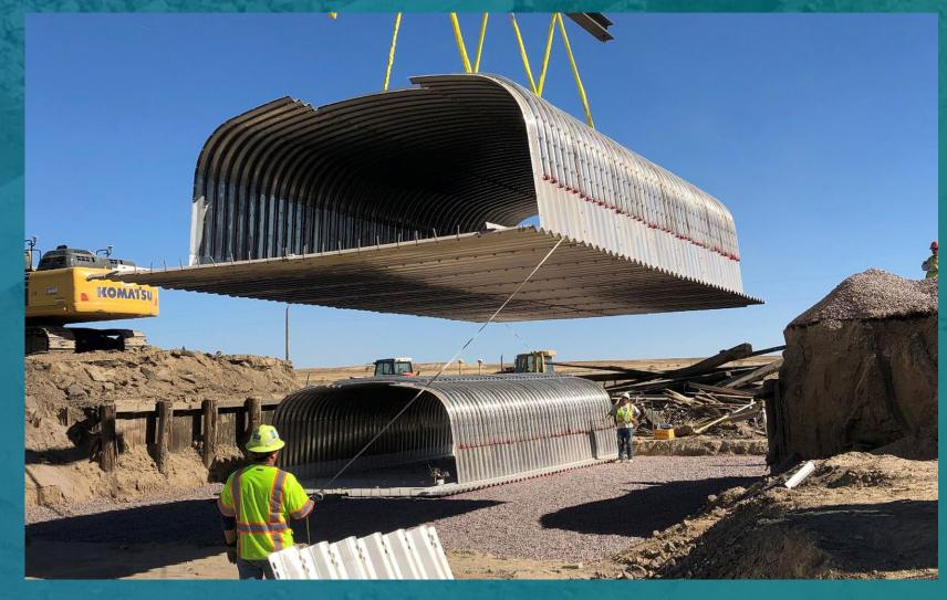
M-21-I – At eight locations, the DB team proposed the use of aluminum box culverts as replacement structures. Aluminum box culverts provided significant cost and schedule benefits and will exceed the intended service life of the structures while minimizing future maintenance costs for CDOT.
