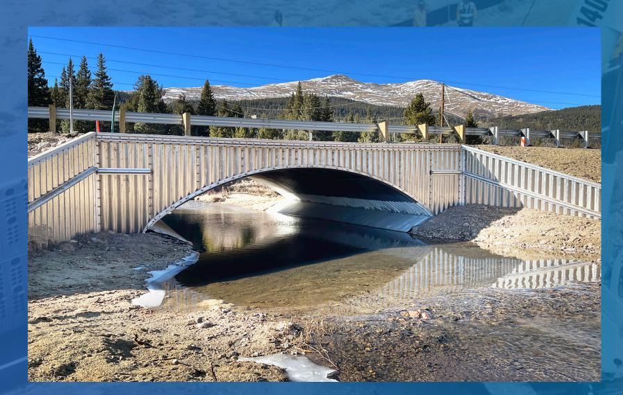
Structure G-12-C – North of Alma on CO 9, the team used an aluminum box culvert with precast, post-tensioned footings and a 7-day highway closure. The team also shifted the structure alignment to avoid wetland impacts while providing lynx migration pathways and fish habitats.
