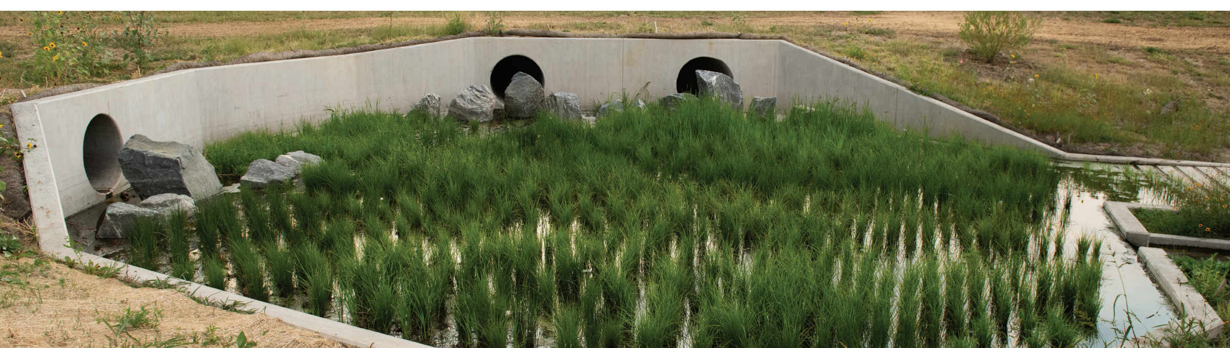
Water quality pond forebays with boulder baffles and vegetated forebays to blend infrastructure with the park's natural environment.
