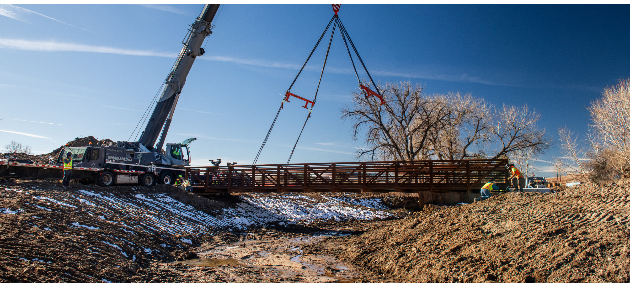
A prefabricated truss pedestrian bridge being placed by a crane.
