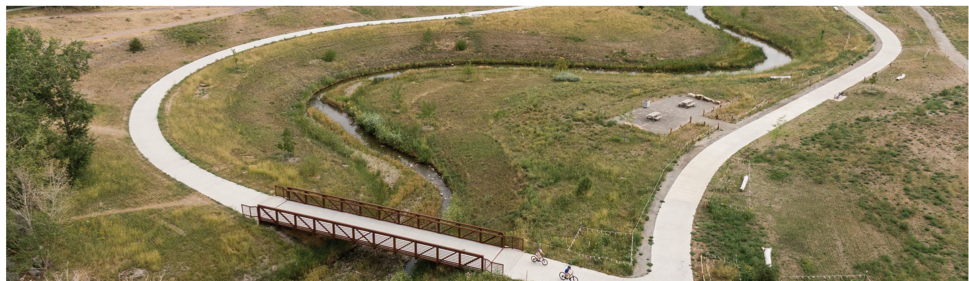
Aerial view highlighting the new pedestrian bridge, trail connection, and channel sinuosity.
