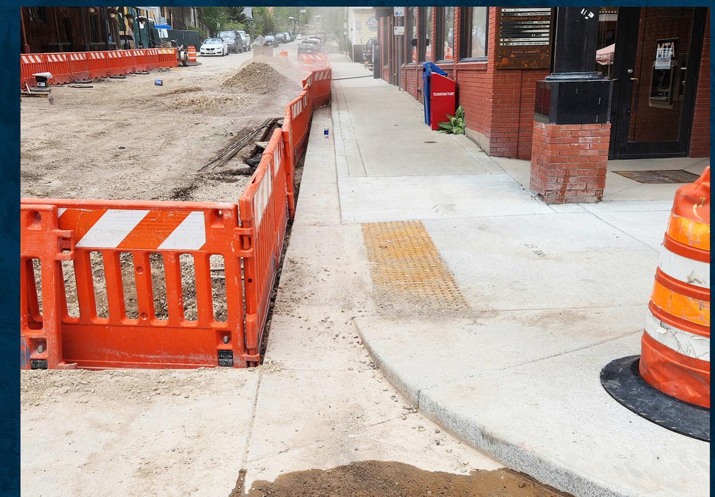
Construction crews reconstruct parts of side streets to improve drainage and new ramp grades.
