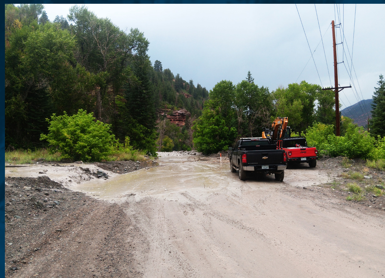
Debris flow at Corbett Creek blocked the roadway, requiring several days of cleanup before reopening.
