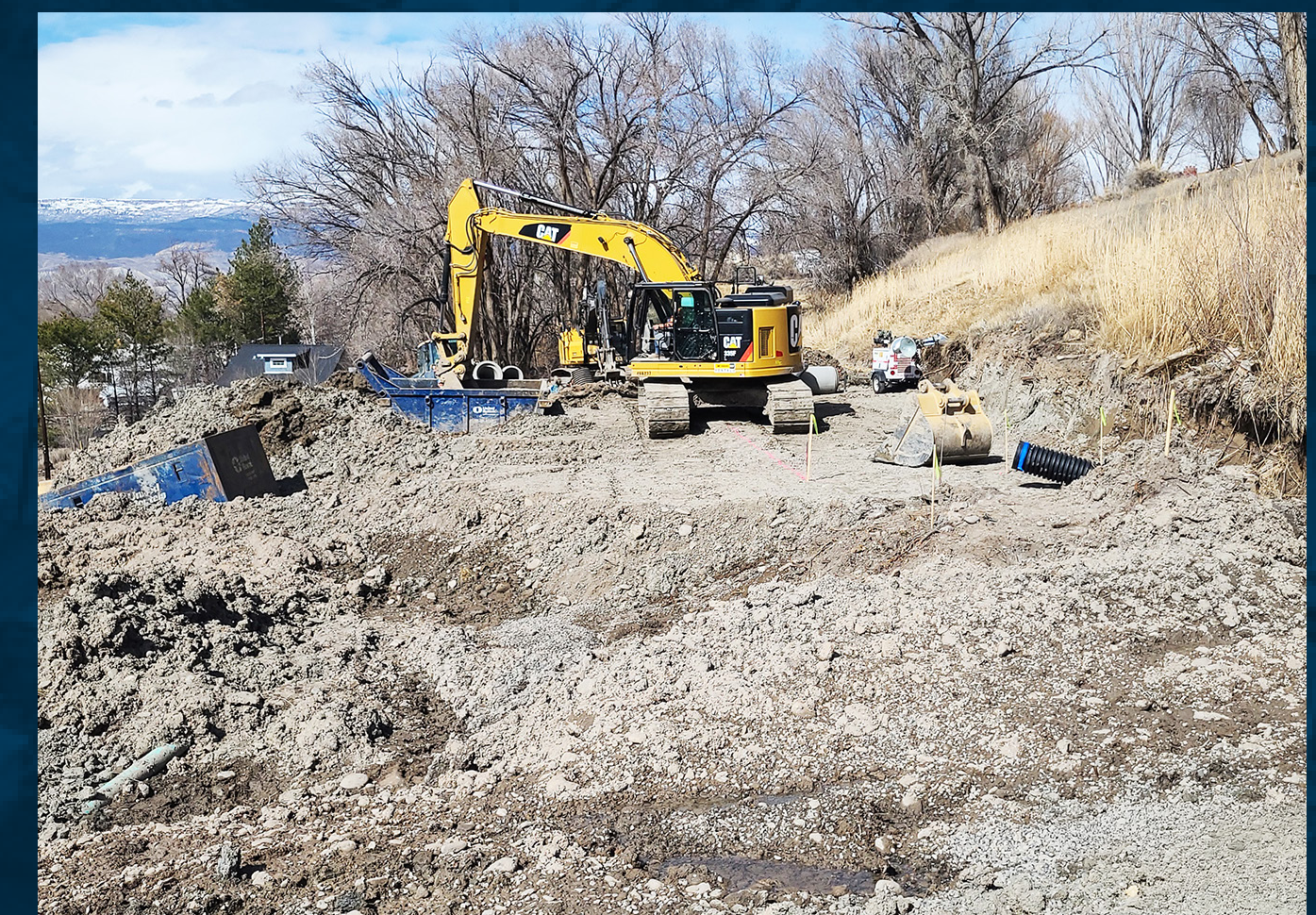
Crews install critical drainage infrastructure above Hillside Street to improve stormwater management and roadway performance.
