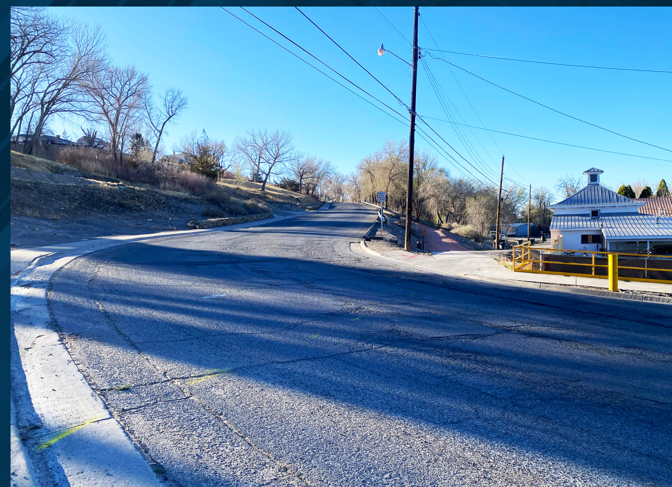
Before reconstruction, steep grades, poor drainage, and limited pedestrian facilities created safety challenges along Hillside Street.
