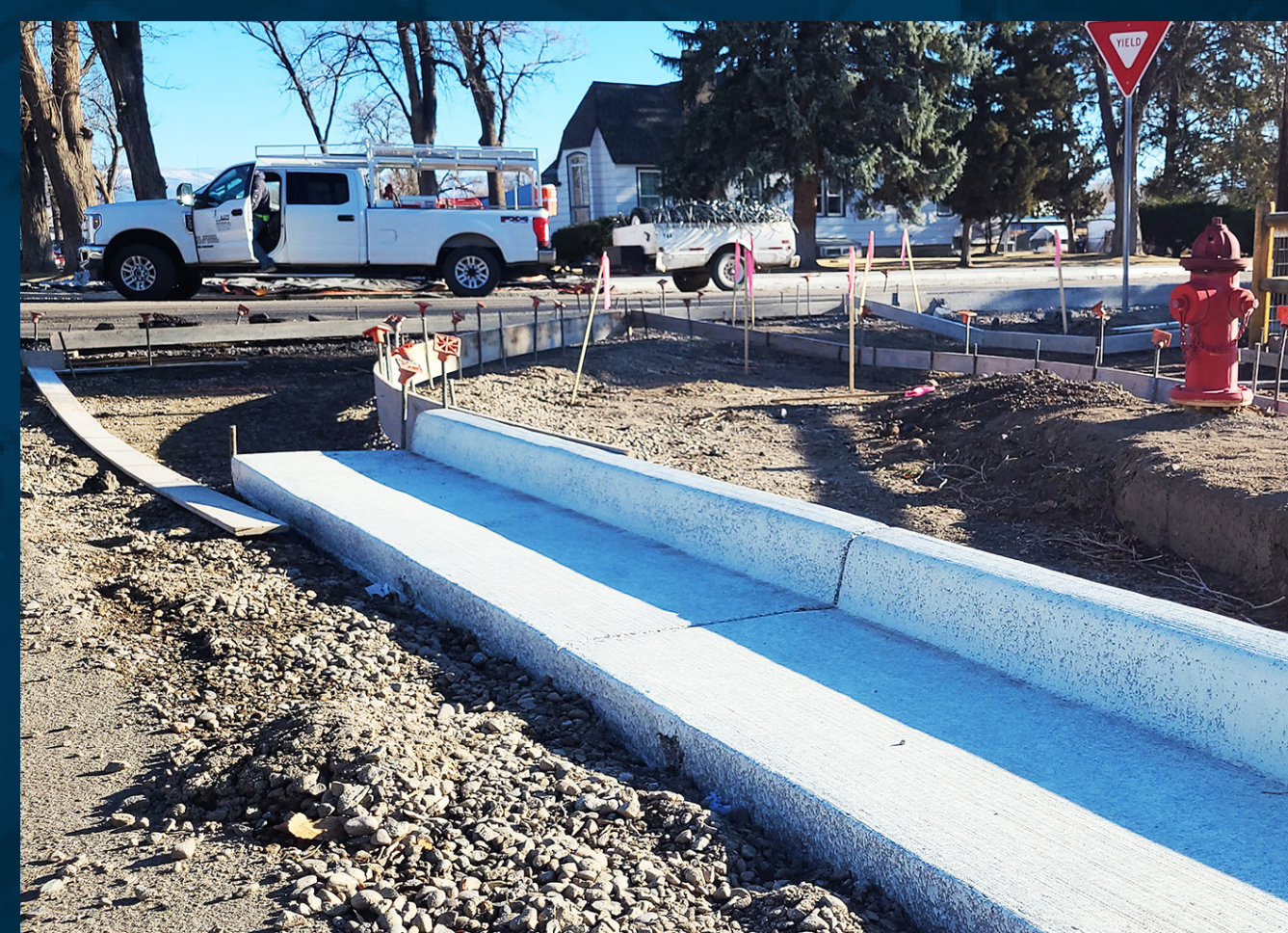
A new pedestrian crossing takes shape, expanding accessibility and improving mobility throughout the corridor.
