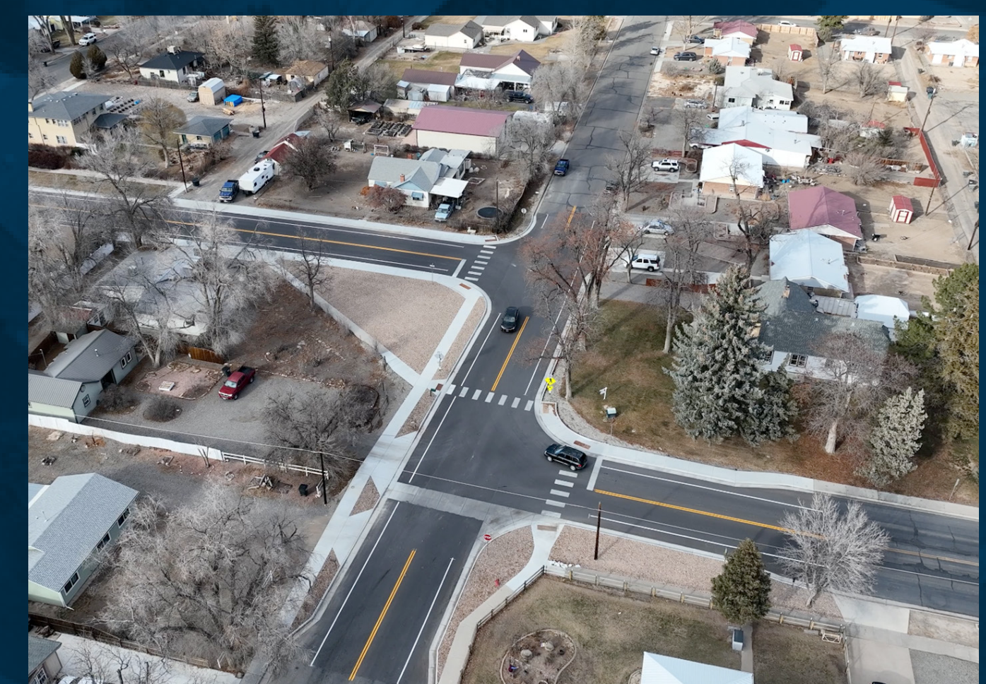
The double-backed-T intersection improves safety and accessibility for people of all ages and abilities.
