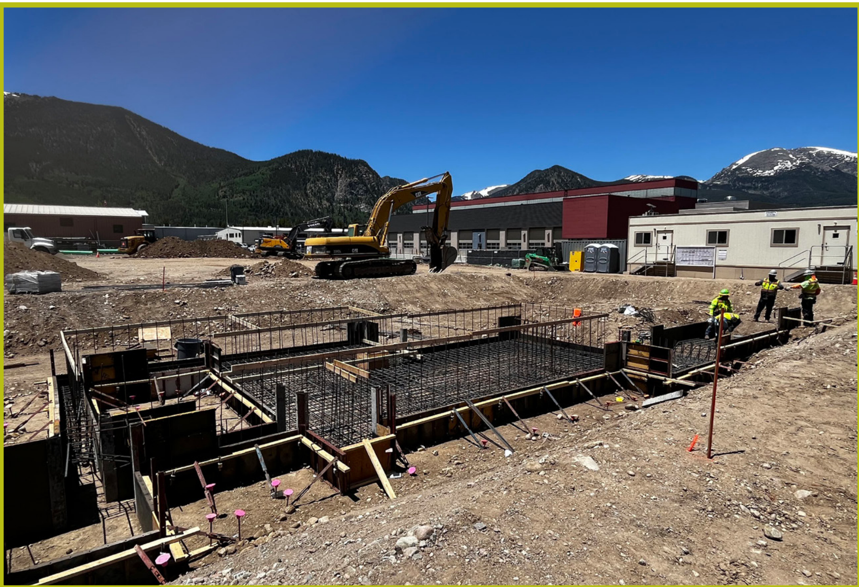
Foundation construction underway at the Summit County Transit facility, where innovative design and infrastructure begin to take shape in the alpine environment.
