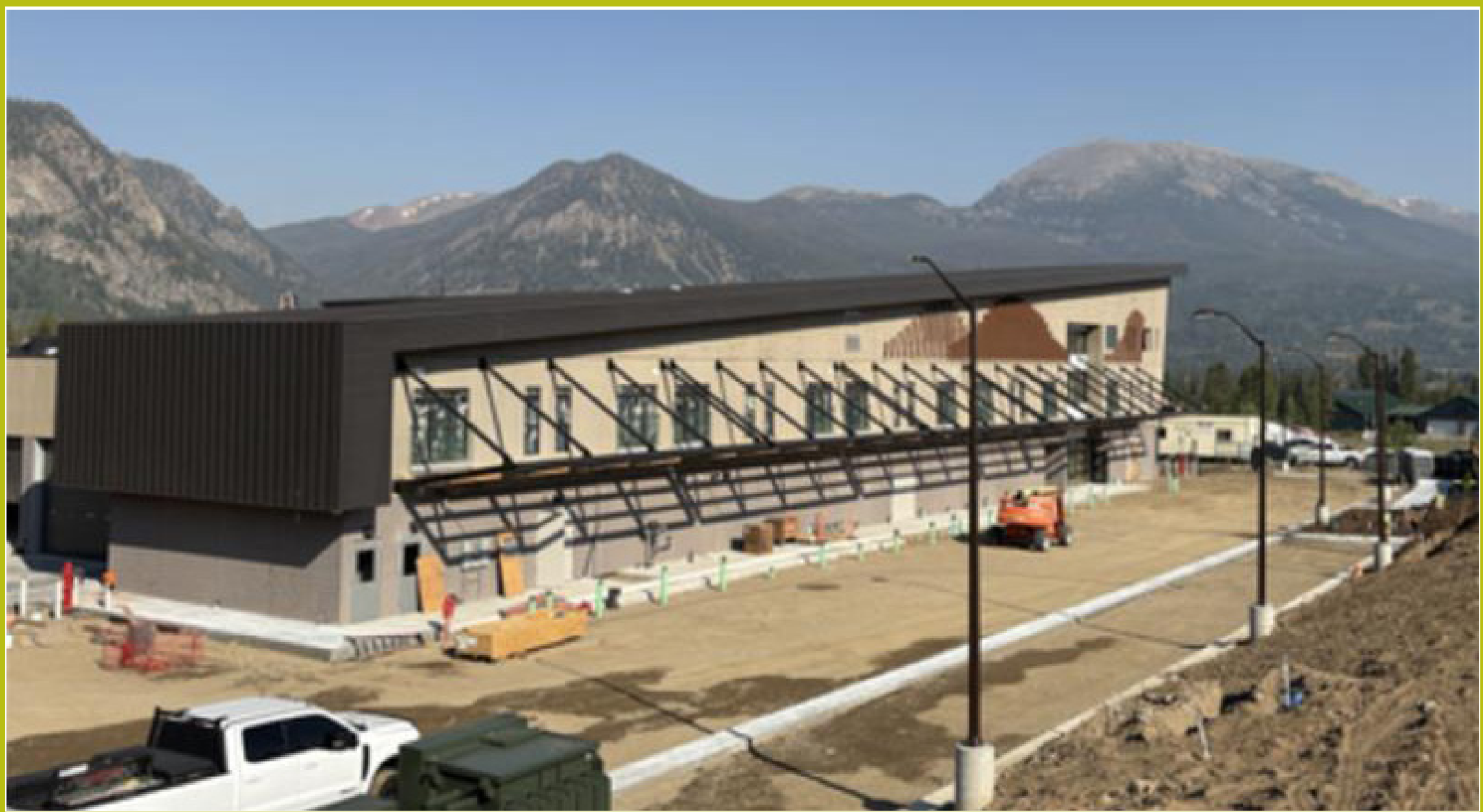
Exterior construction progresses, bringing the facility's distinctive architectural vision into view.
