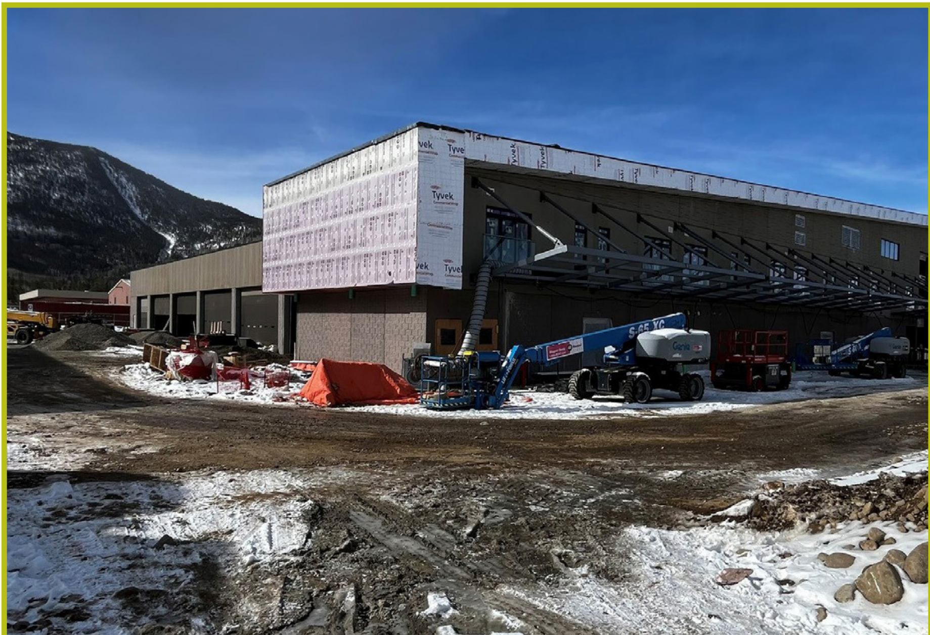
Year-round construction efforts kept the Summit County Transit facility on track despite the challenges of a high-altitude mountain climate.
